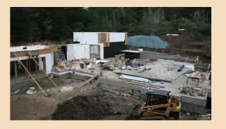
Three concrete mixes have been created to date for the Optimum Performance Home: a specifically engineered Controlled Density Fill (CDF), a standard foundation footing and mix for the Amciv ICF's, as well as a suspended slabon-grade. KIM has been used in every mix except for the engineered CDF.
