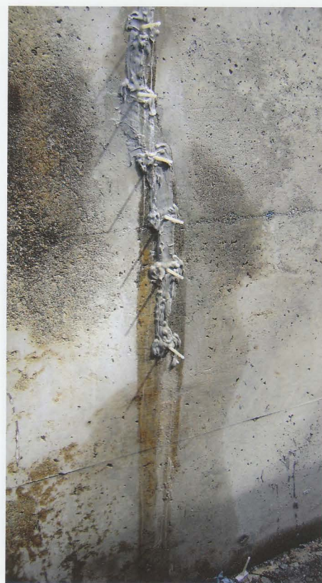
Failed epoxy injection repair
