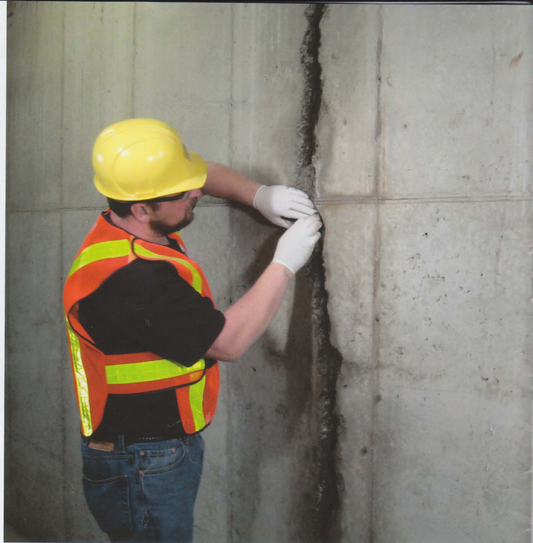
Filling a chiseled chase with crystalline waterproofing.
