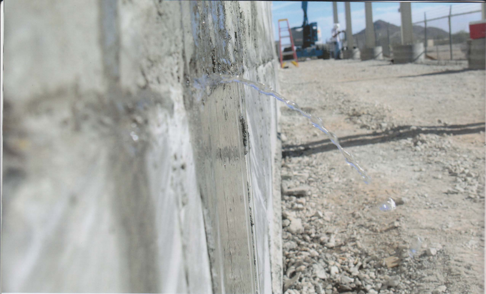
A leaking crack in a fish tank in Arizona, United States.
